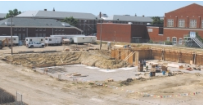
Construction began on the new College of Business building in May 2002.
